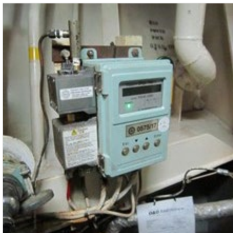
Oily Water Separator
